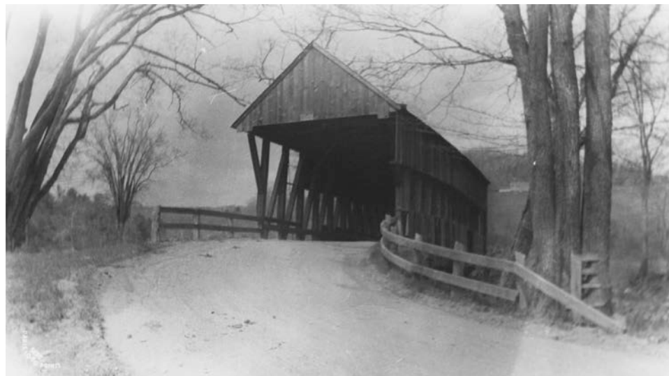
The Clark Bridge, on the west branch of the Ompompanoosuc. This covered bridge, along with Buzzell Bridge and Cook Bridge, were removed as part of the Union Village Dam project.
