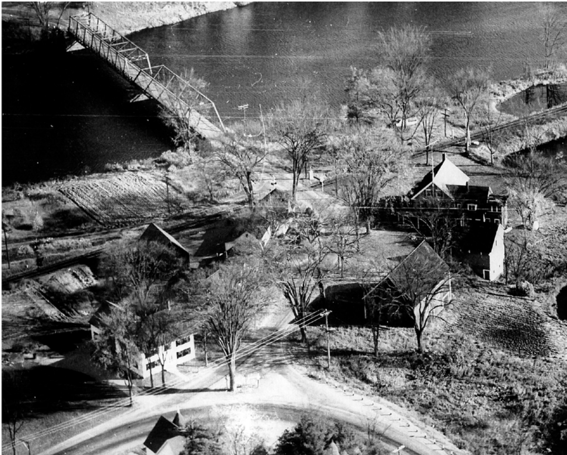
Lyme-North Thetford Bridge, over the Connecticut River. Built ca. 1900, the bridge was damaged by flooding. Only the eastern span was repaired and the western half, weakened, forced closure to vehicles in 1959. With no funds for repairs, the western span collapsed into the river in 1972. Both towns bore the cost, prorated by feet of ownership, of removing the bridge from the river.
