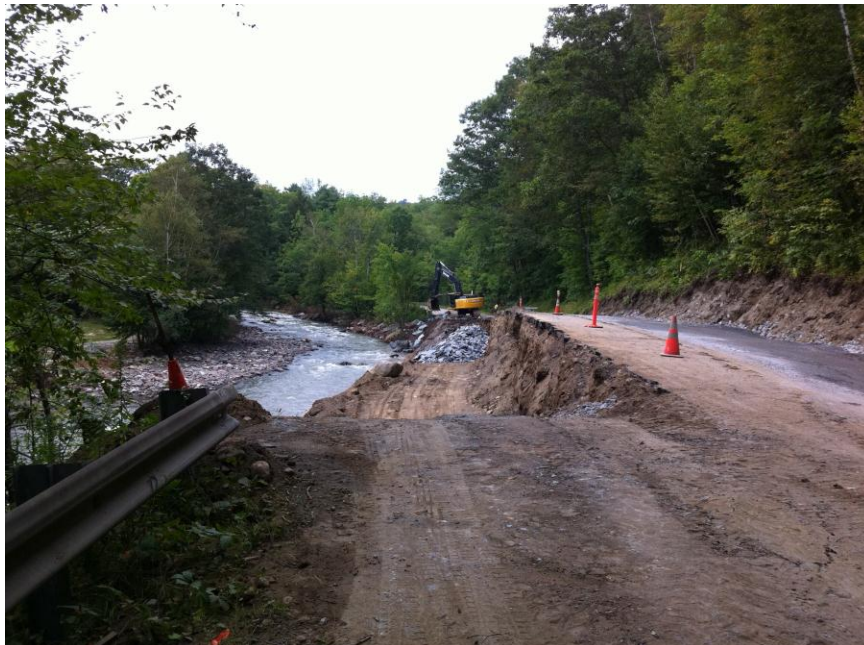
Route 132 Repairs, Day 4
