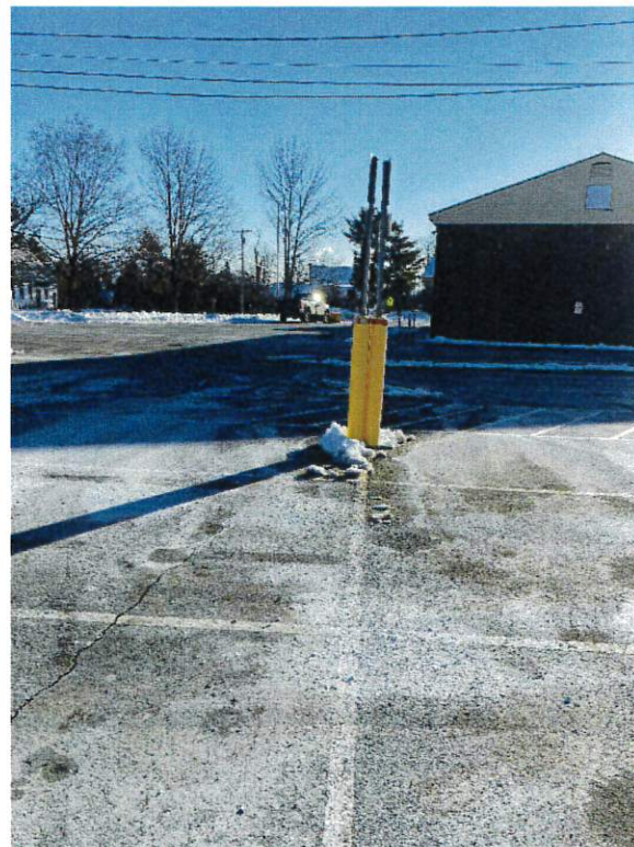
Figure 6: A dual plug EV charging station could be installed adjacent to the ADA parking spaces in the Elementary School lot.
