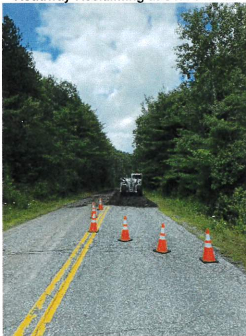
Roadway Reclaiming at STA 340+00
