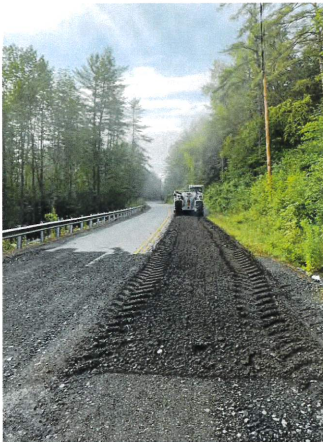
Roadway Reclaiming at STA 314+00
