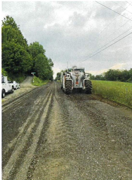
Roadway Reclaiming at STA 303+00
