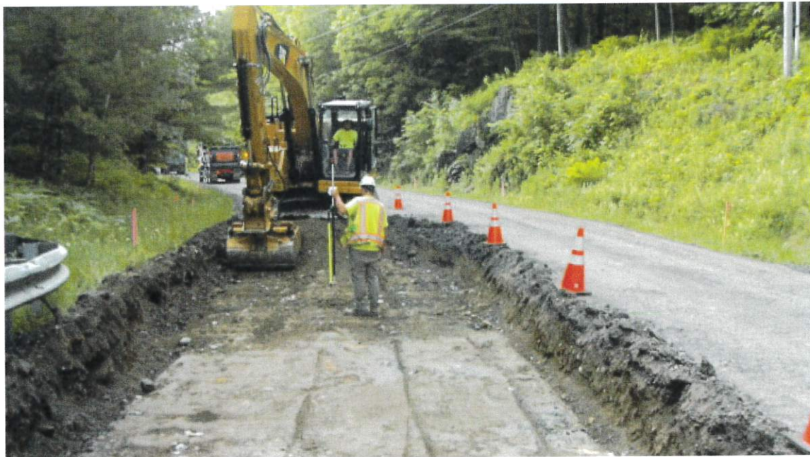
Roadway Box Out
