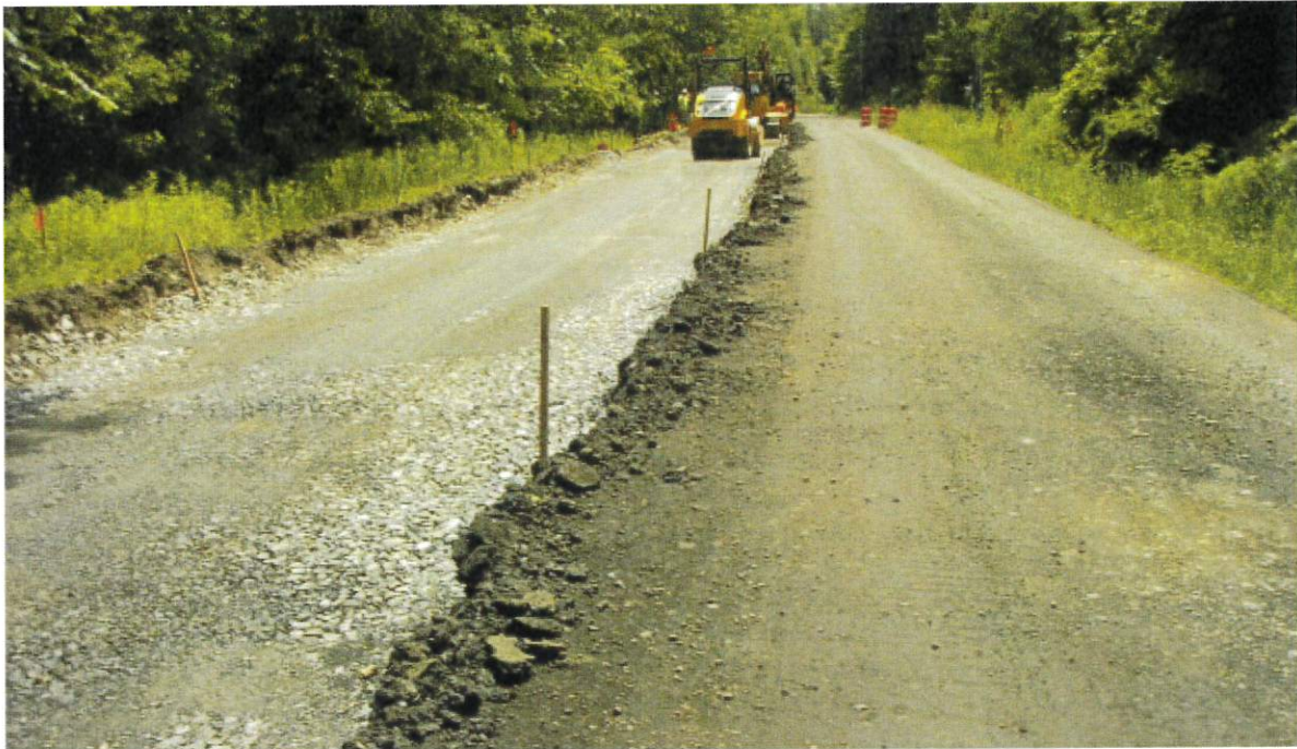
Gravel Compaction
