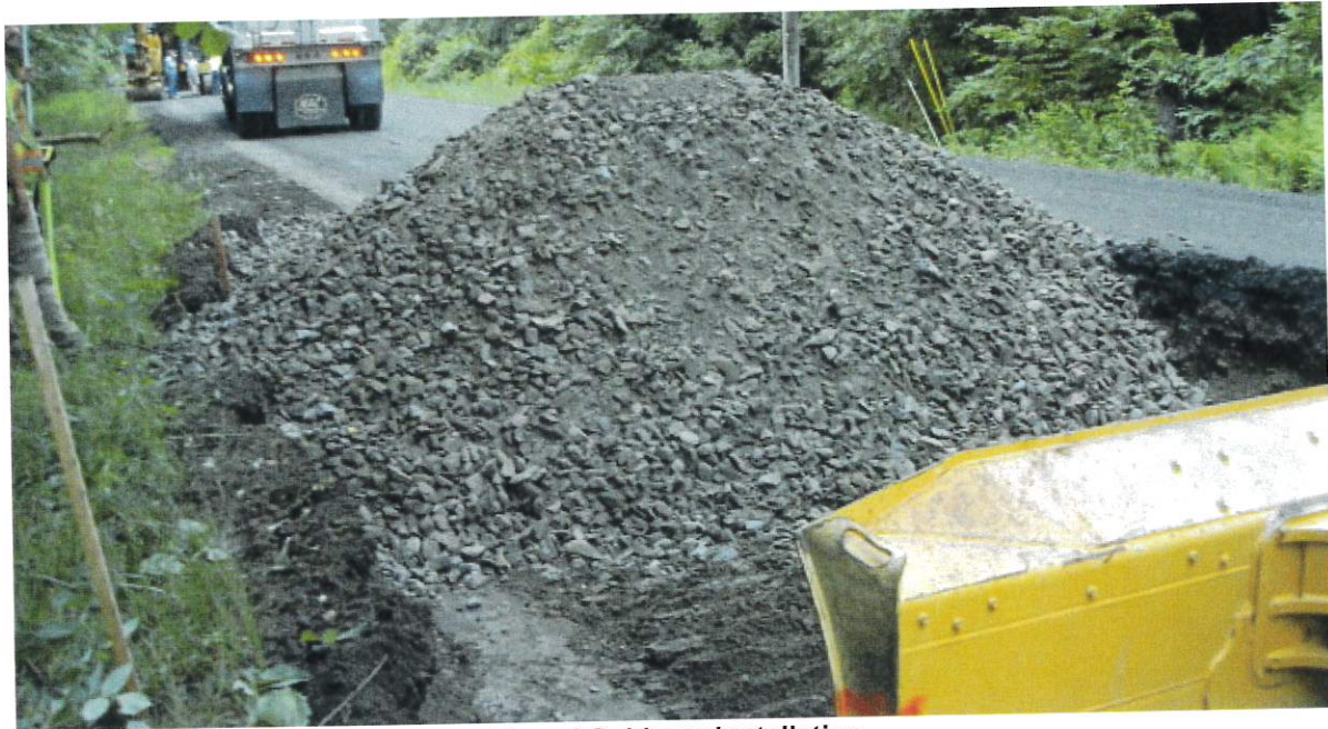
Gravel Subbase Installation
